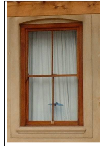
Figure 10: Vertically proportioned window with plastered windowsill and simple plaster-band forming a flat arch above the window.
